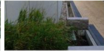
Trincea filtrante - Western Harbour, Malmö
